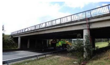
Case study C2 (PC girder bridge)
